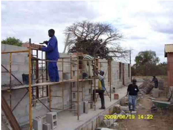
Erecting the rear wall of the building
