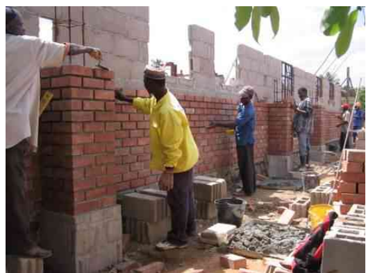
Starting the brick face on the south side of the hospital
