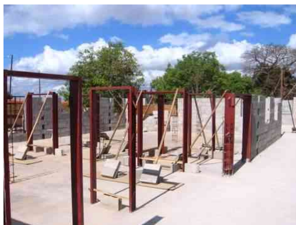
The future surgical block awaits the block layers
